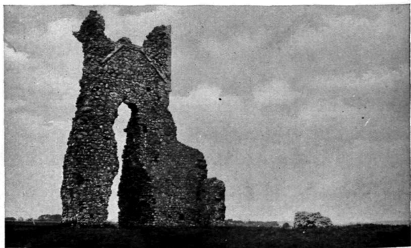
Fig. 8.—EASTBRIDGE from South-East.
